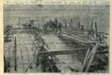
Fig. 25.—Casting Concrete Arch. Rings.
